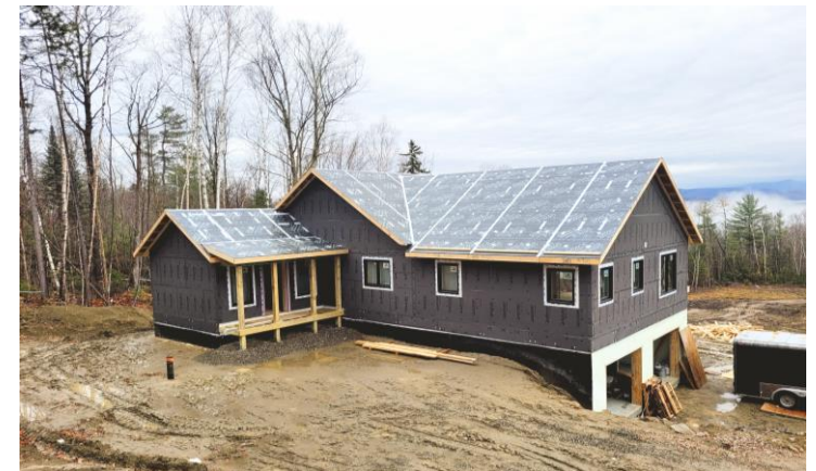
Completed OPA home
