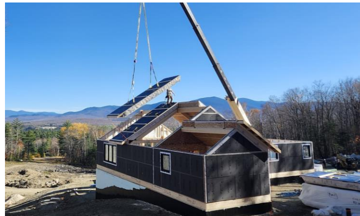
OPA panels being installed
